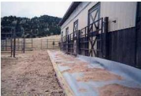
After working on the French drain, I wanted to keep the horses from kicking the shavings out of their stalls onto the sand. I cut a 4" x 2" board the exact width of the door and with screws attached some rubber matting so that it would stick up a few inches. The horses don't kick this 2" x 4" out of the way because it fits tight right up to where the door frame sticks out. I would like to try the type of brush found on the inexpensive snow scrappers instead of the rubber sometime.
